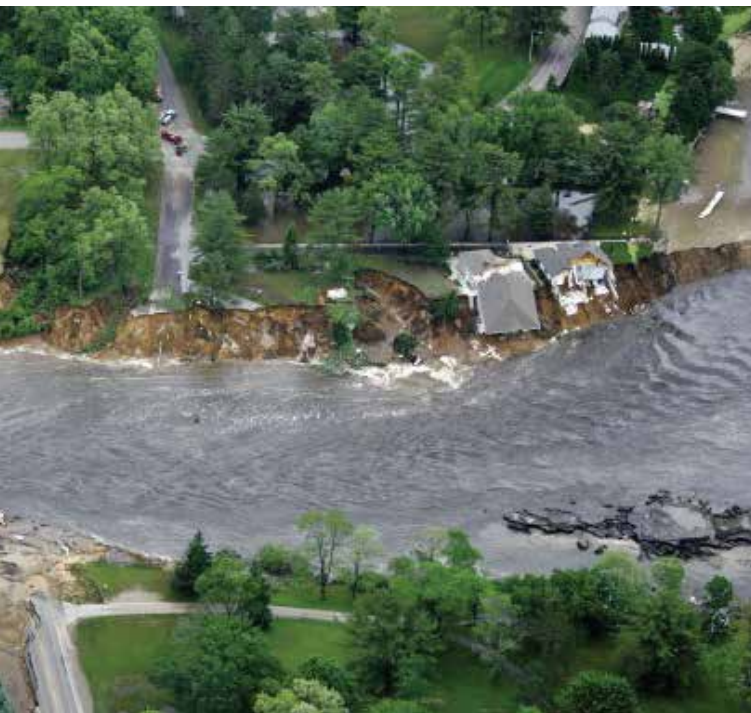
During the 2008 flood events in Sauk County a shoreline of Lake Delton collapsed, draining the lake into the Wisconsin River, destroying homes, and severing a county highway. Photo by Madison Newspapers.
